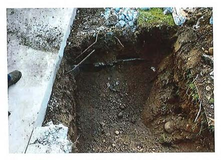
Looking east at UST #2 pit area following removal. Note water line on east end of pit.
