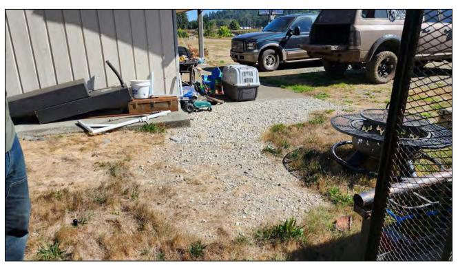
$Photograph\ 2.\ Gravel\ backfill\ at\ location\ of\ former\ USTs\ near\ southeast\ corner\ of\ house.$
