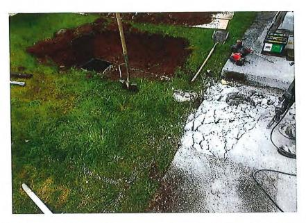
Looking west at UST #1 exposed for removal and concrete removal over UST #2.
